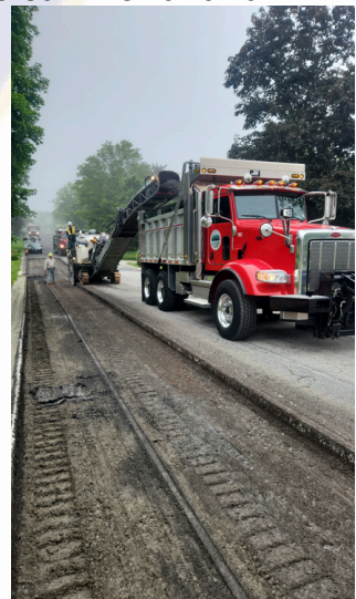
Mt. Pleasant Township, helping with Twin Lakes paving project.
