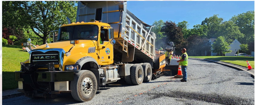
Cumberland Township Maintenance Department working on Twin Lakes paving project.
