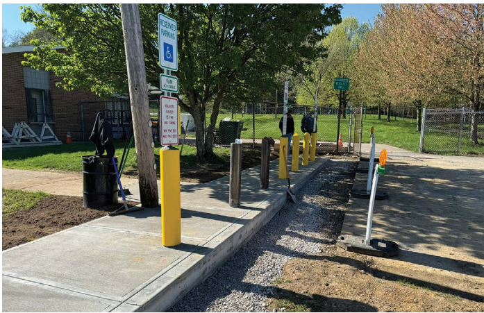
New handicap parking spots – concrete was installed by Public Works
