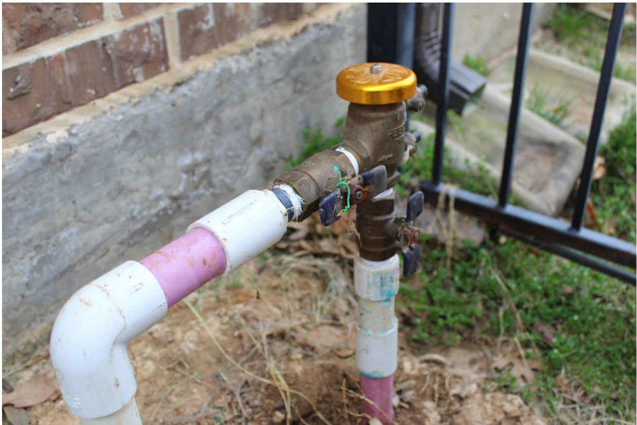
Example of above ground PVB backflow prevention assembly
