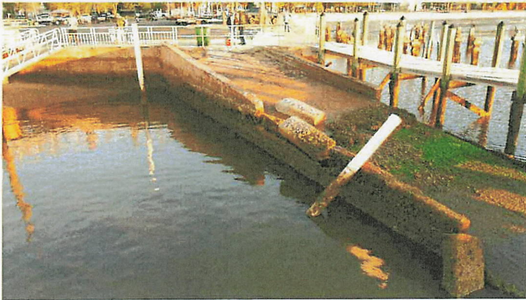
Old ramp next to current launch ramp may require demolition based on the results of the planning and design study conducted as part of this project
