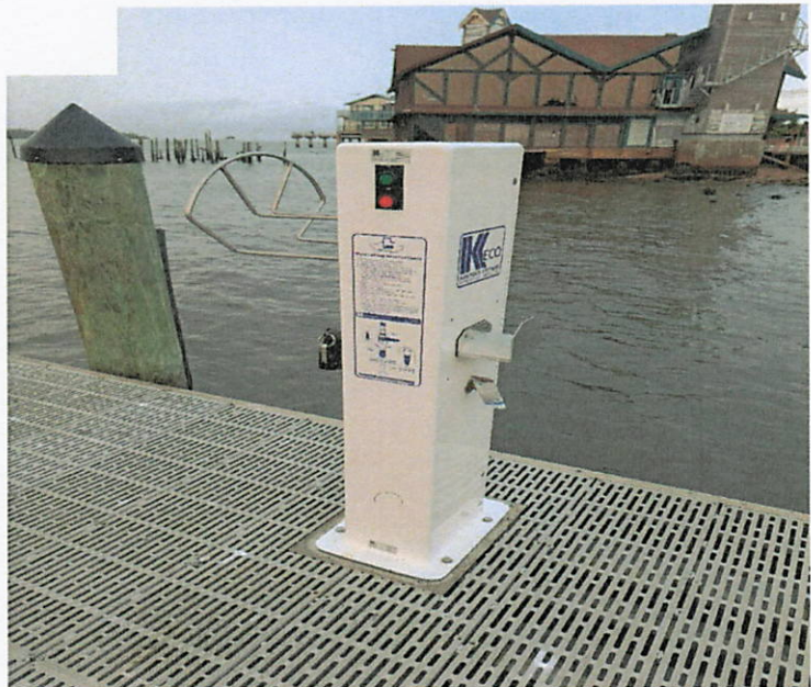
Pump Out Station on Fixed Dock
