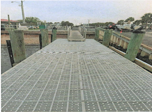
Fixed Dock and Composite Decking
