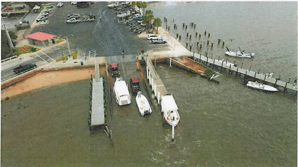
Narrow ramp makes simultaneous launch difficult. This is an example of combined commercial and recreational launching.
