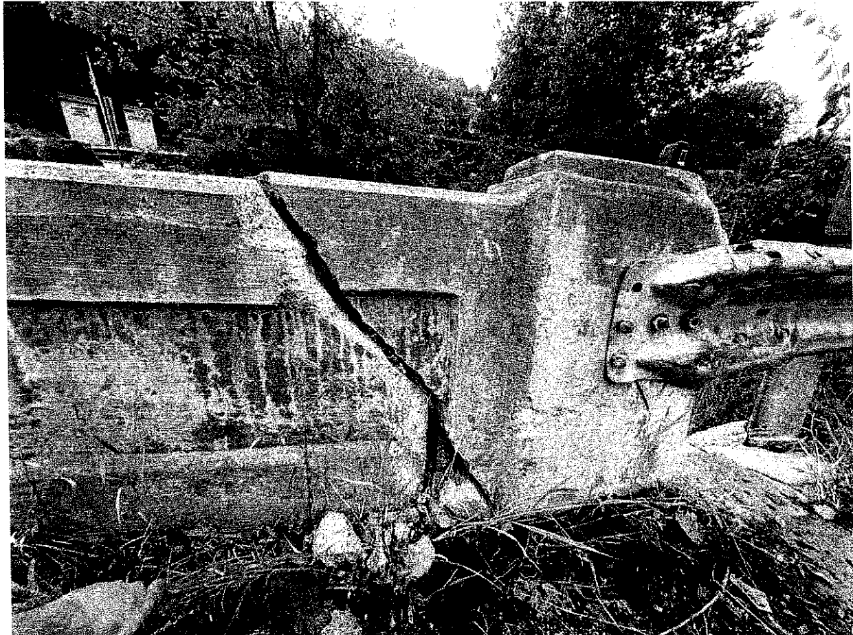
Photo 2: The near right bridge barrier patch exhibits collision damage for 4' L. The collision caused the barrier to breakoff and shift, only held in place by the rebar within the barrier. Barrier may not contain and/or redirect an errant vehicle.
