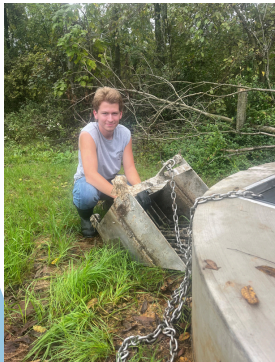
Chase cleaning out the debris basket of a manhole
