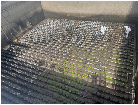
South Plant tank cleanout
