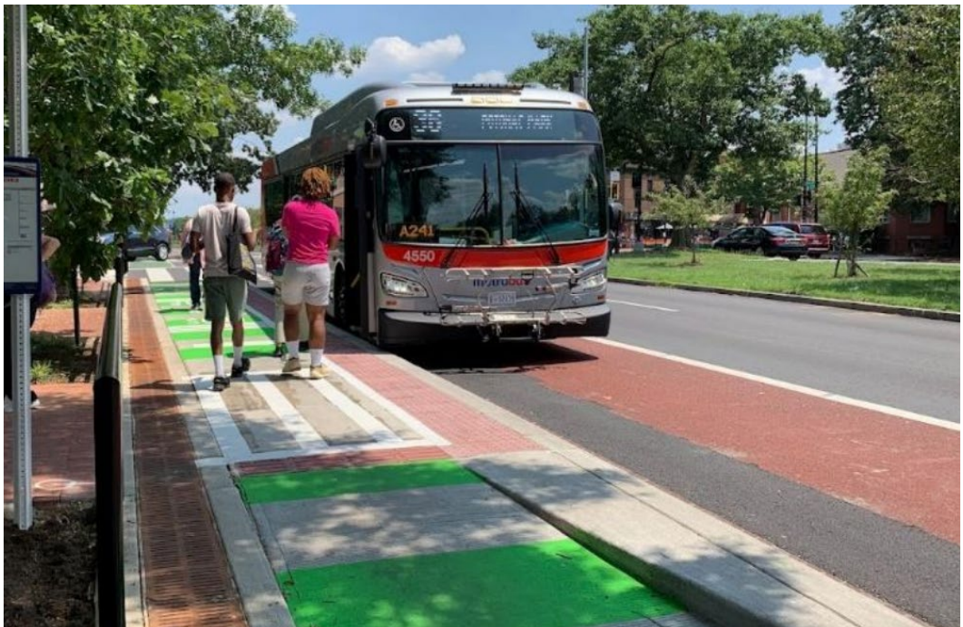
Example of ramped elevated bus loading pads
