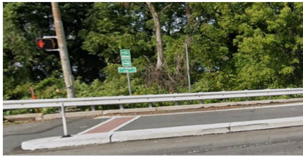
Front Street Shared-Use Path in Harrisburg, PA
