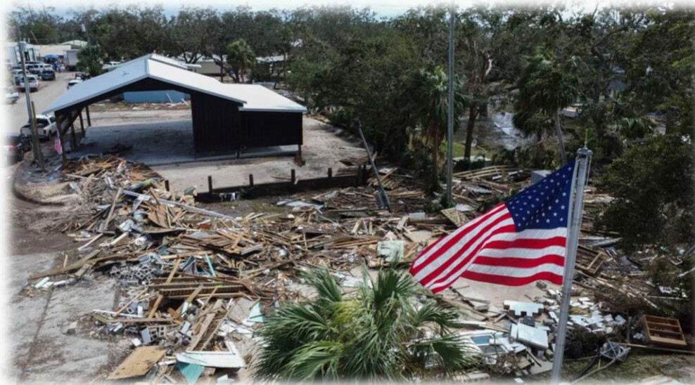
Where decisions were once made, only debris remains. Hurricane Helene didn't just damage a building — it displaced the heart of the community. Even in destruction, the Town's resilience stands stronger than the storm.
