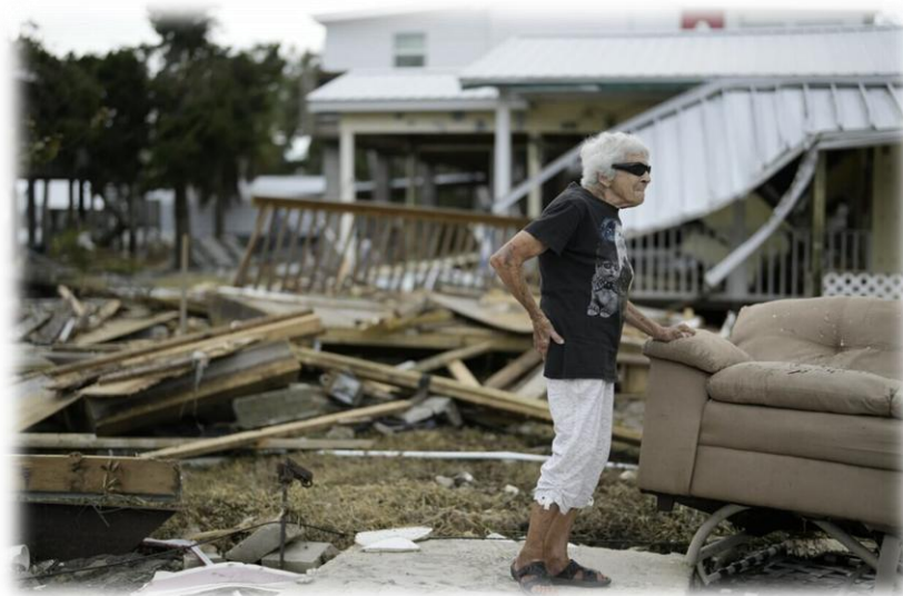
Hurricane Idalia (August 30, 2023). Storm surge and wind destroyed more than 75 homes and damaged public infrastructure across the Town.
