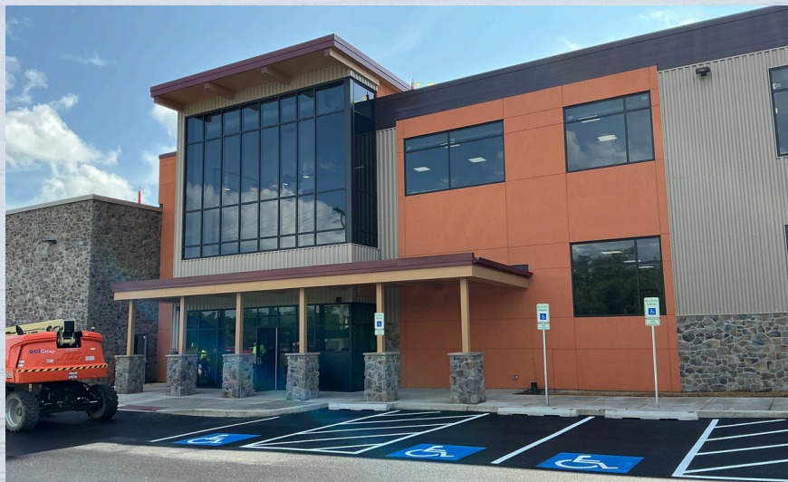
Front Entrance of New Building Addition Project 08/24/26
