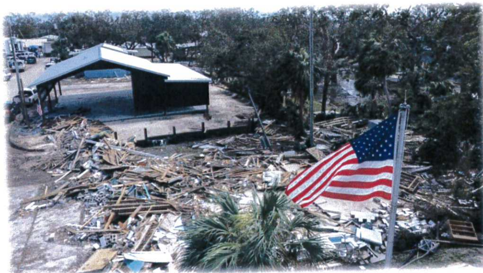
Where decisions were once made, only debris remains. Hurricane Helene didn't just damage a building — it displaced the heart of the community. Even in destruction, the Town's resilience stands stronger than the storm.
